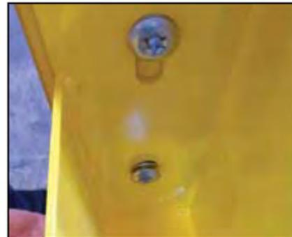
Optional field installed fasteners.
